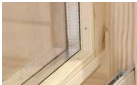
Real glass windows and doors, single glass or double glazing
